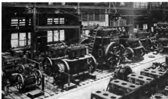
Multi-Cylinder Gas Engines on Testing Floor
